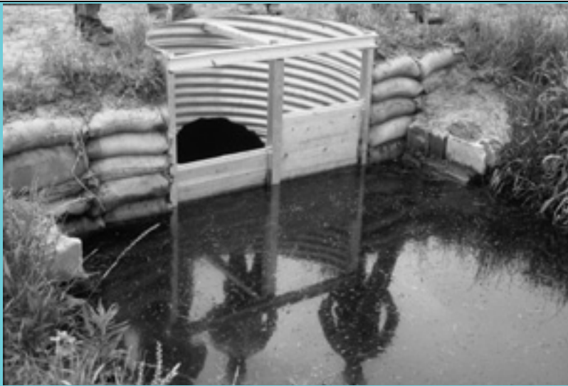
Fig. 2 Controlled drainage system showing flashboard riser ( http://www.soil.ncsu.edu/ )
